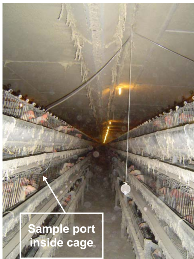
Figure 4: Sampling lines and aisle sensor for manure-belt (MB) house.
