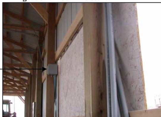
Key to labels: A=enclosure and location of wireless data transmitter (Wi-box)
