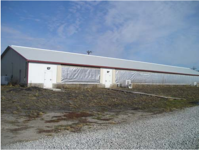
New gestation breeding barn with solid waste separation.
