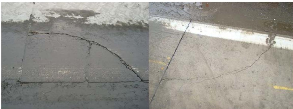
**Figure 9. Corner breaks on both side of the cell 32 concrete slab**
