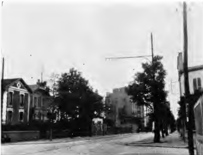
A plain street in a suburb of Paris, which shows the way the French run wires behind the street trees, and prune them to the rear if required; and how the trolley poles set in line with the trees hardly show at all.
