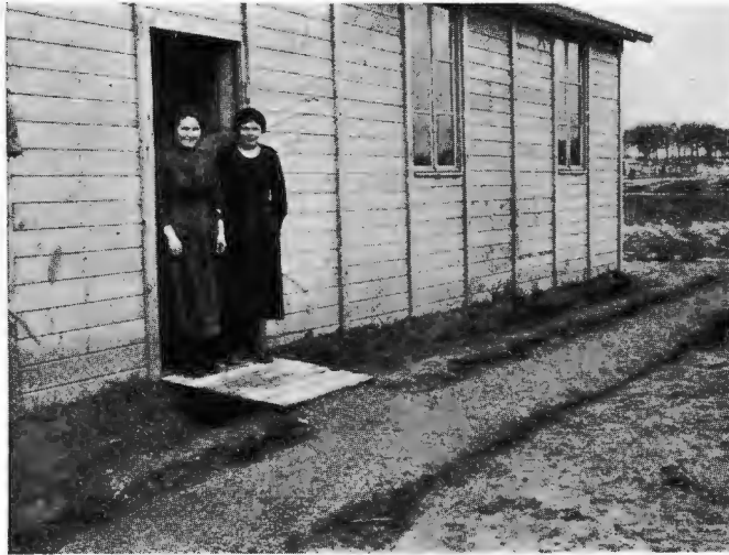
Barracks at Allerey, showing how the panel construction enabled the armies to use small trees and short boards, and to have the panels made up standard anywhere,—in France, Switzerland, or Spain, to be erected when needed and moved if required. French chamber maids.
