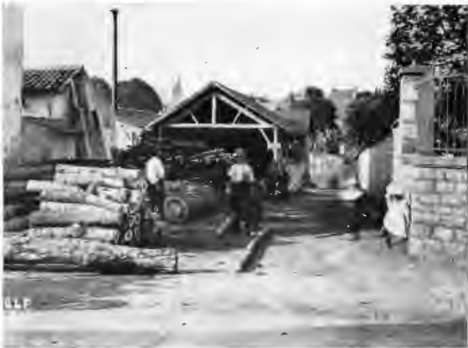
Village sawmill at Verdun-sur-Doubs. Typical of most of the country. Larger places have larger mills on the same plan. Some logs are rafted and a few shipped by rail, but most of the lumber supply of France is hauled by horses direct from the forest to the mill, and is used in the commune where it is sawn.
