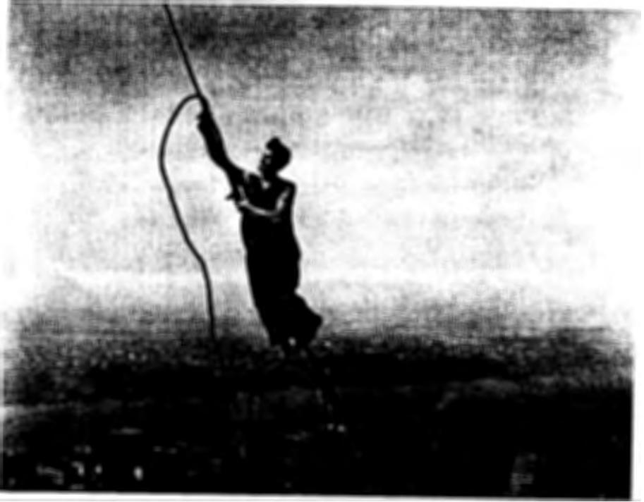
Lewis Hine's photograph, *Icarus*, showing a worker fastening steel cable to hold a derrick in place prior to lifting steel girders and other steel parts at the top of the Empire State Building. (Bettmann/Corbis)
