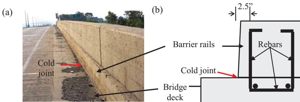
**FIGURE 1.** (a) A photograph of a highway overpass showing the cold joint between the road deck and the barrier rail. (b) A schematic showing the locations of rebars that anchor the barrier rail to the bridge deck.
