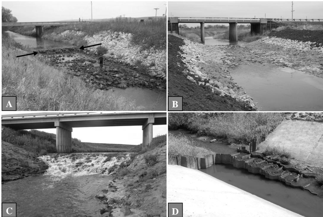
Figure 1. A) Sheet pile weir with loose riprap slope, originally built at 1:20 (rise/run), but note how rock has moved away from the sheet pile weir (black arrows). B) Sheet pile weir with 1:20 grouted riprap slope. C) Sheet pile weir with 1:4 grouted riprap slope. D) Sheet pile weir with 1:20 fish ladder and steel baffles.
