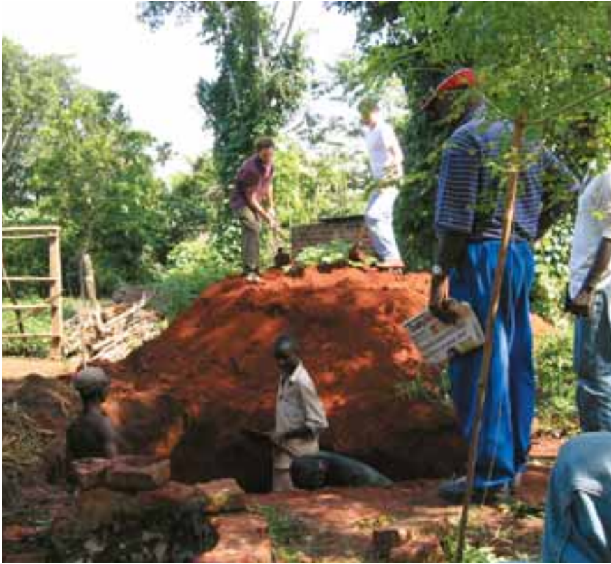
...and then work with Ugandans to dig a pit for the digester.
