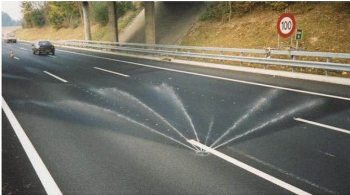
Figure 5 - Boschung FAST - Fixed Automated Spray Technology (Boschung 2013b)
