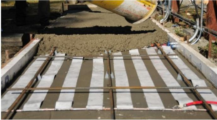
Figure 4 - Construction of conductive slab with carbon fiber tape (Yang, et al. 2012)
