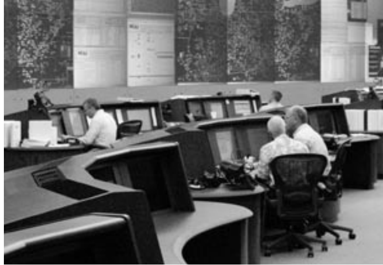
Photo courtesy of Midwest Independent Transmission System Operator, Inc., Carmel, Indiana— www.midwestiso.org
