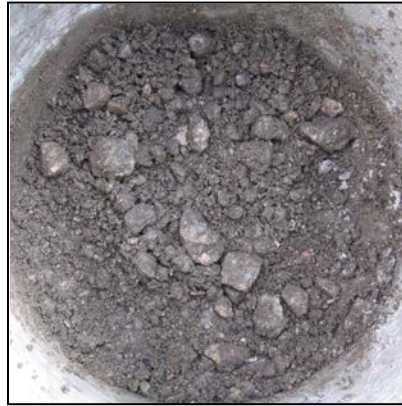
Figure 1. RCA subbase condition underneath concrete slab after coring.
