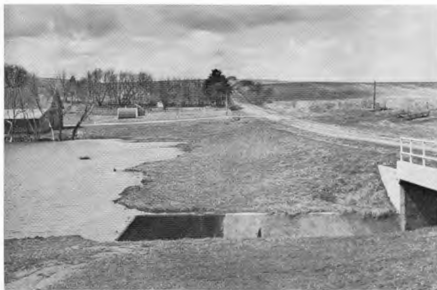
This reservoir—like most western Iowa reservoirs—probably loses about an inch of water a day through seepage. Agricultural engineers are testing various chemical treatments to reduce this seepage loss.
