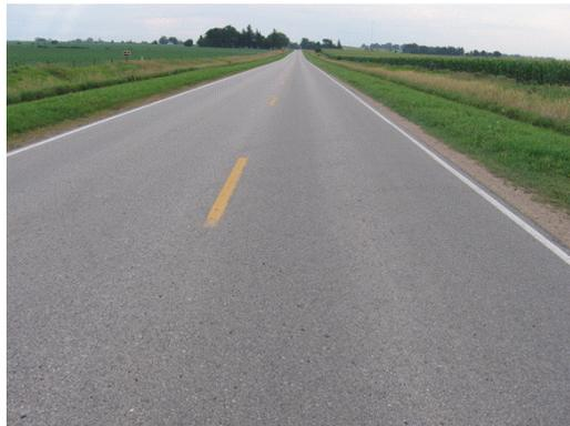
Figure 8. Picture of distress-free HMA surface on rubblized PCC (test section no. 4: C23 in Franklin county).
