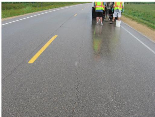
Figure 9. Picture of longitudinal cracking on HMA overlaid rubblized PCC (test section no. 3: IA3 in Delaware county).
