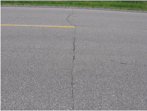
Figure 10. Picture of low-temperature cracking on HMA overlaid rubblized PCC (test section no. 1: D16 in Blackhawk county).
