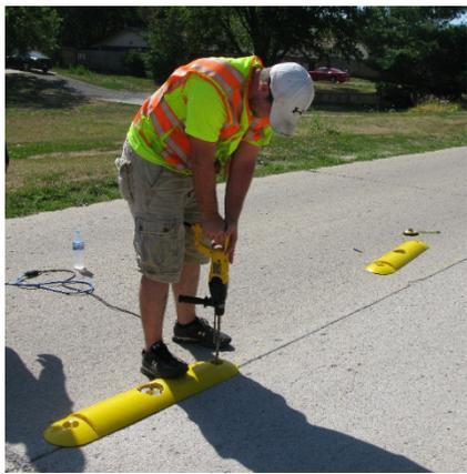
*Installation of raised curbing using bolts*
