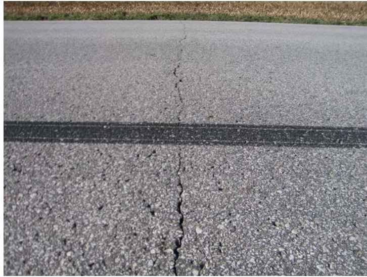
Fig. 8. Picture of low-temperature cracking on AC-overlaid rubblized PCC pavement (No. 3: D16 in Black Hawk County)
