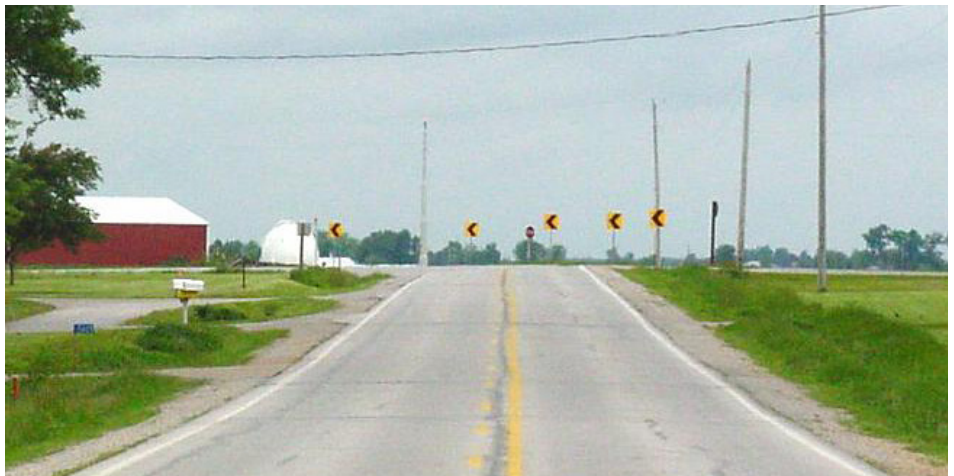
Figure 1. Oversized chevrons on US 6 in Johnson County, Iowa (Tom Welch, Iowa DOT)
