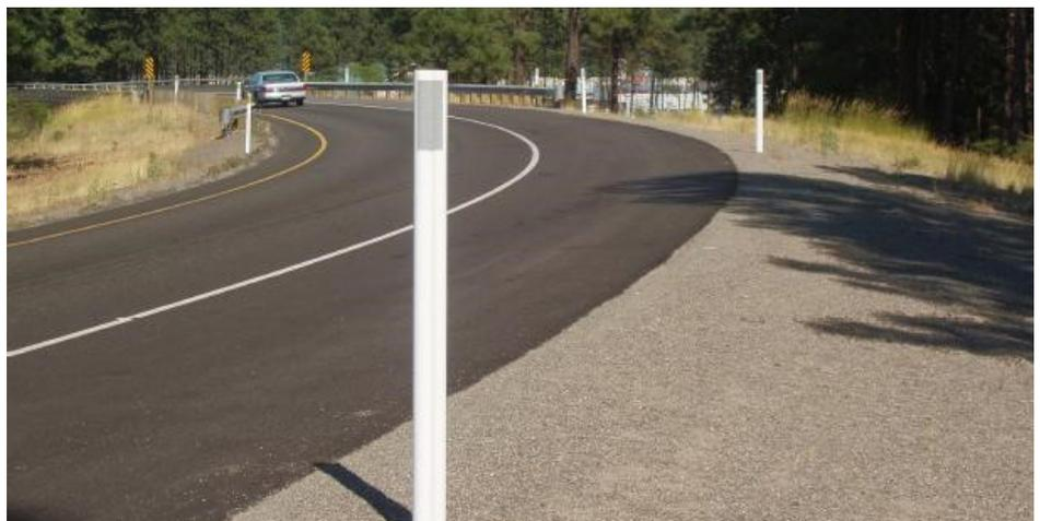
Figure 1. Delineator posts along a curve (© PEXCO)
