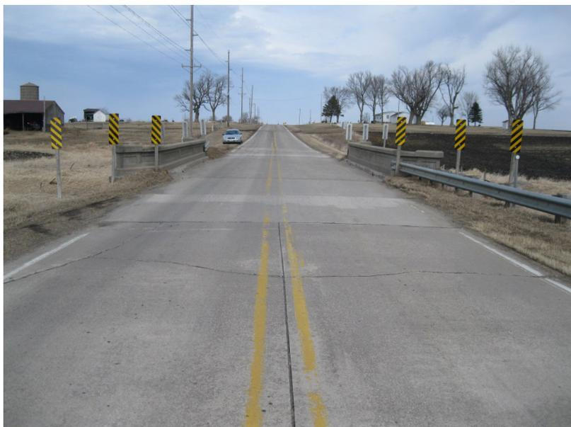
Rural Iowa farm-to-market road that has concrete bridge deck in fair condition with numerous pits and popouts, spalled and crumbling fascia, and steel girders in satisfactory condition (Image: Bridge Engineering Center)
