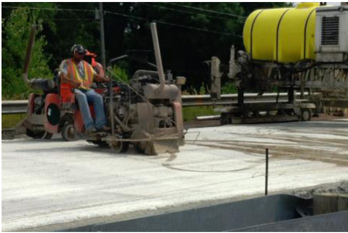
Typical conventional saw-cutting process
