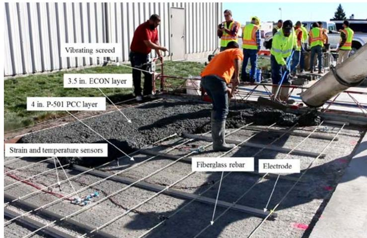
**Figure 3. ECON HPS construction procedure at DSM**
