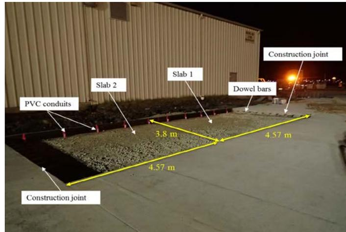
**Figure 2. ECON HPS construction location at DSM**
