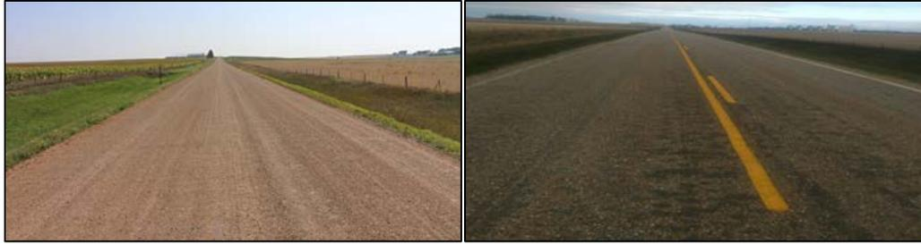
**Figure 3. Appearance of Otta seal at immediately after the construction (left) and one month post construction (right).**
