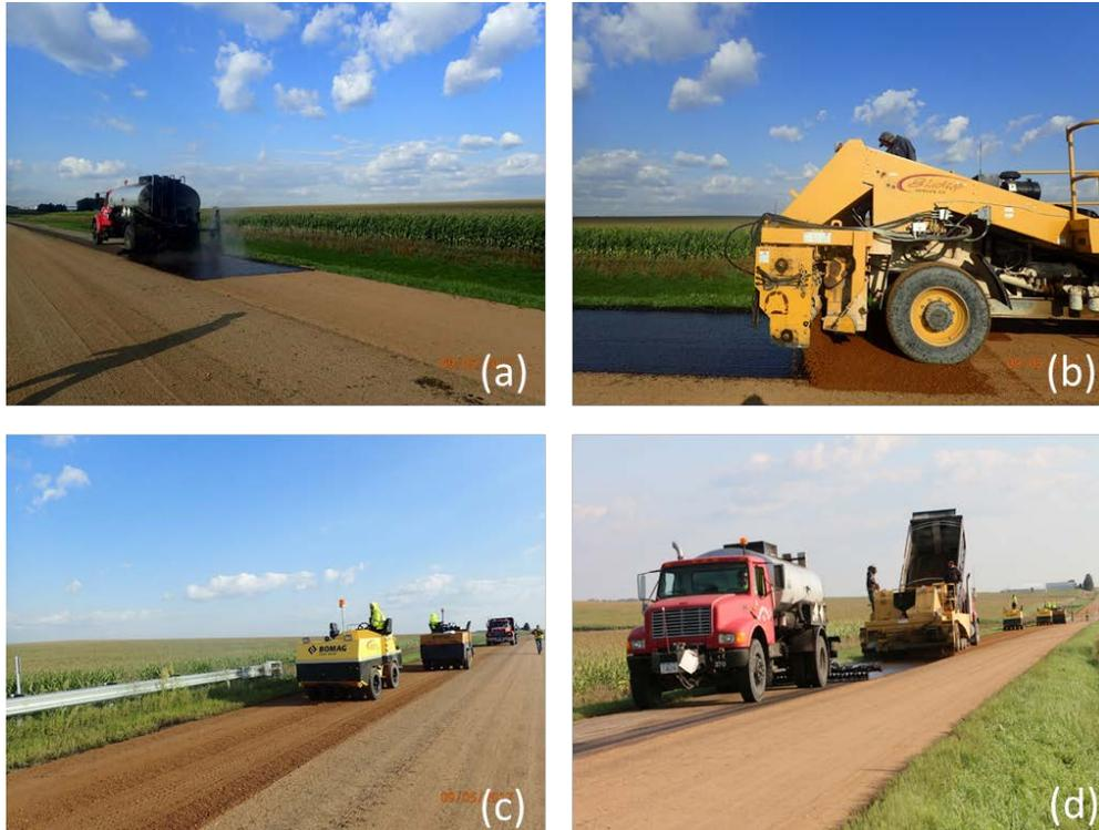
**Figure 2. Otta seal construction process of (a) binder spraying, (b) aggregate application, (c) rolling compaction, and (d) the complete process.**
