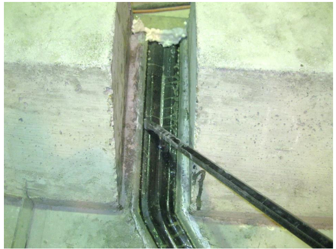
Use of a crowbar to install D.S. Brown gland
