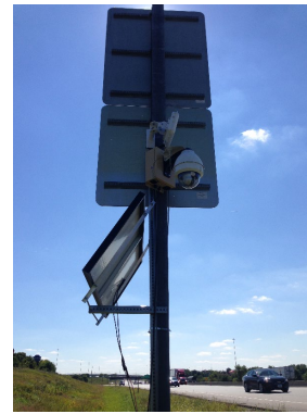
Figure 1 Camera and side-fired radar sensor installation
