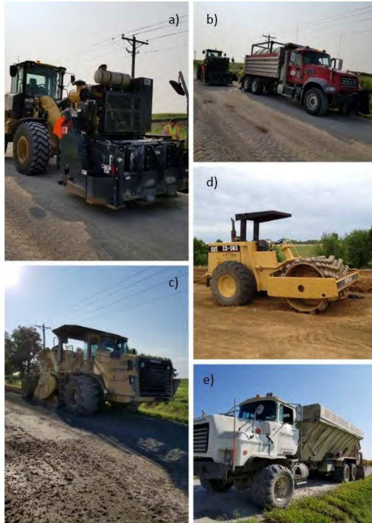
**FIGURE 2** Equipment used for chemically stabilized sections: (a) RoadHog reclaimer; (b) water truck with chemical stabilizer added to tank connected to RoadHog; (c) road reclaimer; (d) sheepfoot vibratory compactor; and (e) powder spreader truck.
