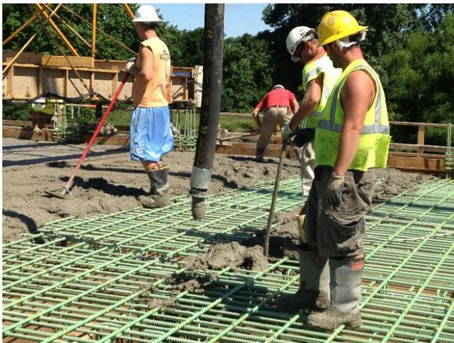
*LWFA concrete placement on the bridge deck*
