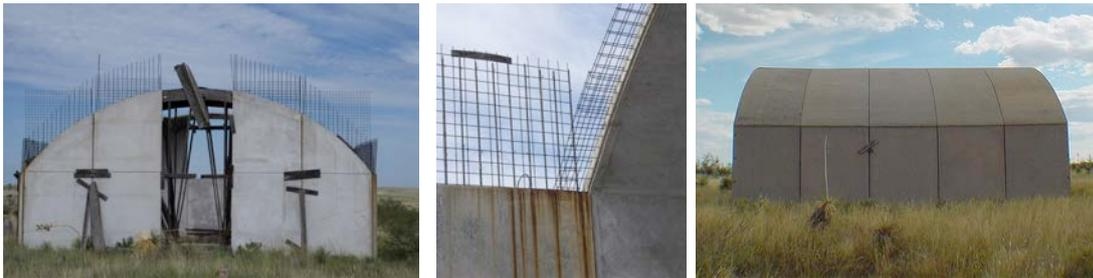
Figures 9A-9C: (Left to Right), The unfinished building with temporary bracing and roof panel formwork in place, the wall / roof intersection showing the modest reinforcing sizing, and a side elevation of the finished building showing sagging in the roof and deflection in end walls.
