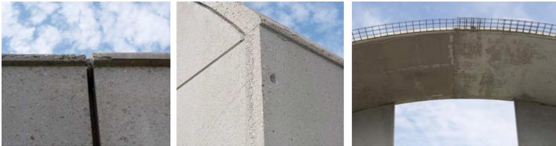
Figure 10A-10C: (Left to Right), Concrete broken at the roof edge, poorly crafted reveals at outside corner showing evidence of sandblasting on the surface, & a view of the underside of the roof showing the difference in quality in the concrete between the walls and the roof.
