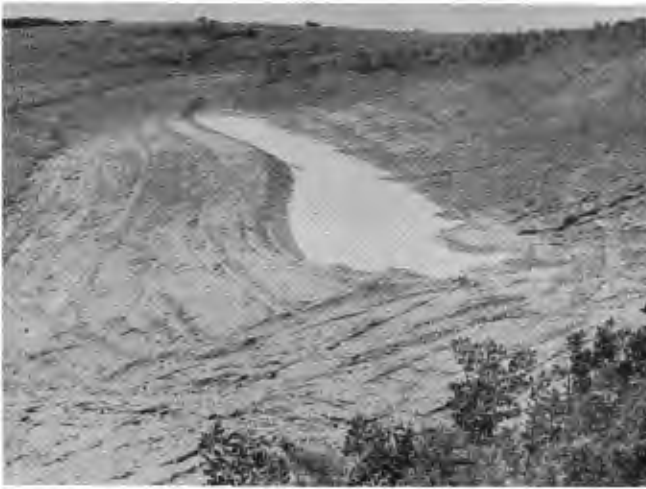
Basin terraces are built to protect farmland against the runoff from steeper slopes above. But it's necessary to establish vegetative cover on the areas disturbed by construction. Note rilling on the unprotected area at left. Researchers at Iowa State are trying to learn more about the fertilizer requirements for establishing and maintaining cover. Notice the unfertilized area in photo at right.
