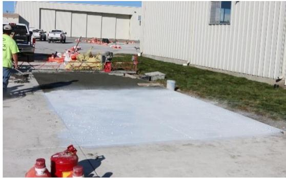
**Figure 1. Construction of two ECON HPS test slabs at Des Moines International Airport, November 2016**
