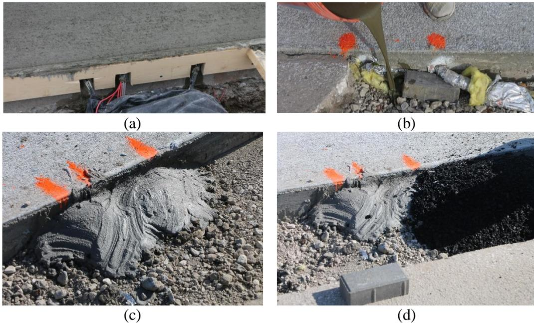
**Figure 3. Images of the wires and the protection layers utilized in the IA DOT project: (a) sensor and power wires imbedded in ECON layer, (b) preparation for pouring hot mix asphalt concrete, (c) additional concrete layer to provide structural support, and (d) hot mix asphalt covering the protected wires**
