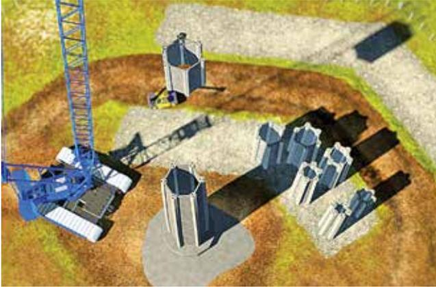
**Figure 4.** Assembly of a Hexcrete tower using preassembled cells.
