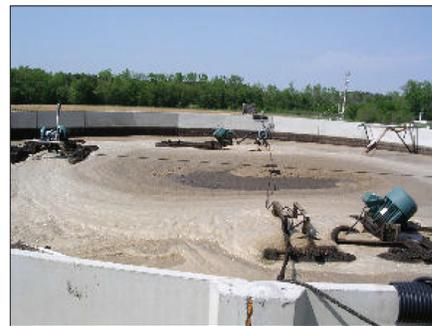
Figure 1. Surface aeration units and mixers in a concrete swine manure storage.
