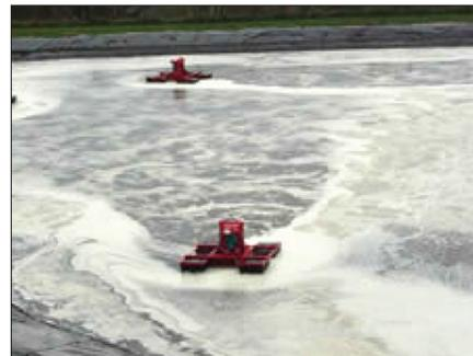
Figure 2. A floating aeration unit. In this unit, air and manure are mixed in a vortex as it passes through the pump impeller. Discharge is below the fluid surface to encourage oxygen transfer.
