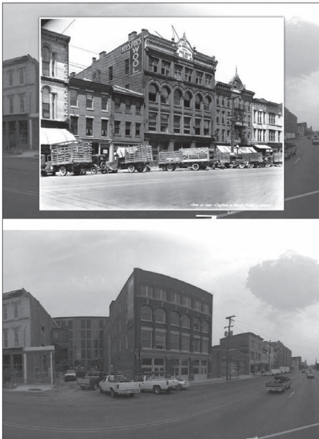
Figure 3: 1933 photo of a building compared to modern Google Street View of the same building.
