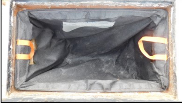
(a) interior of non-proprietary CBI
