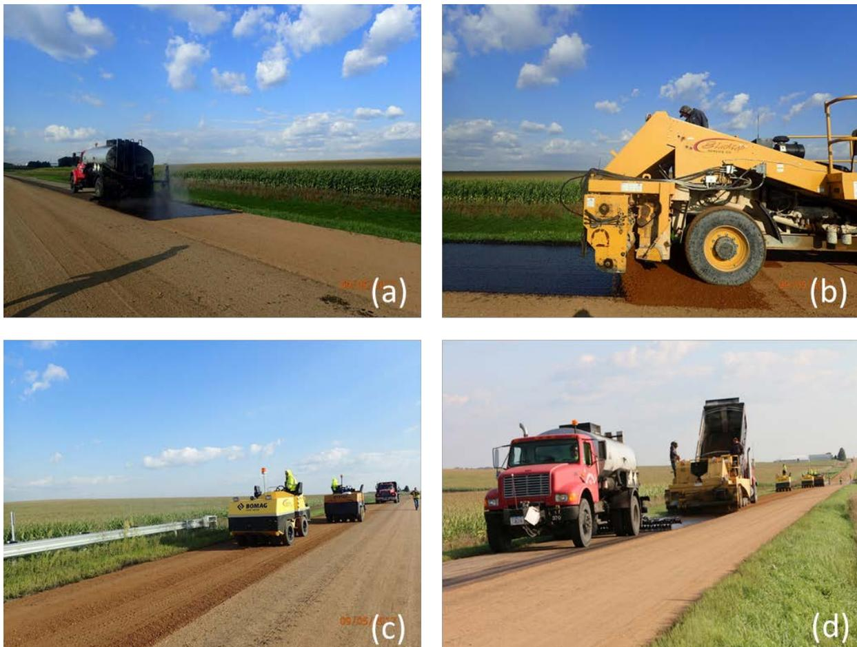
**FIGURE 3 Construction of Otta seal: (a) binder spraying, (b) aggregate spreading, (c) rolling compaction, and (d) the complete construction process.**
