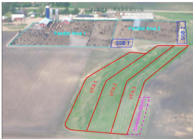
Figure 2. Layout of Central Iowa 1 and the VTS used to control and treat runoff generated by the facility.
