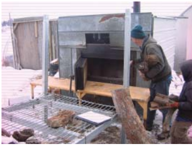
A Working Group mini-grant enabled Greg Hoffman to add a wood burning boiler to his small vegetable/fruit farm and heat a hoop house to extend the growing seasons.
