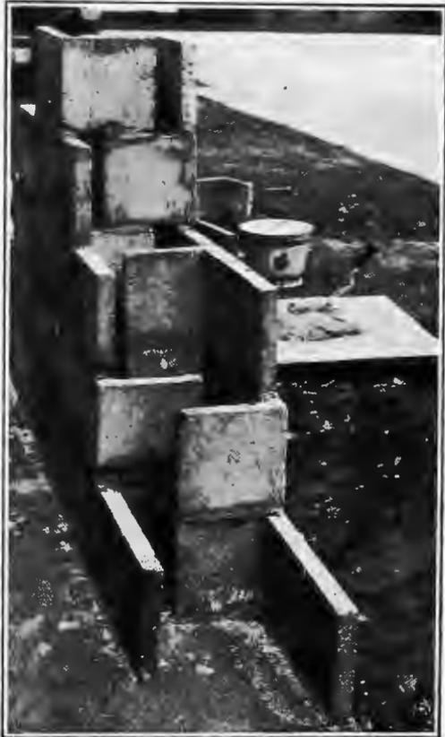
Fig. 14. There is little opportunity for the transmission of moisture or the conduction of heat in a wall laid up in this manner.
