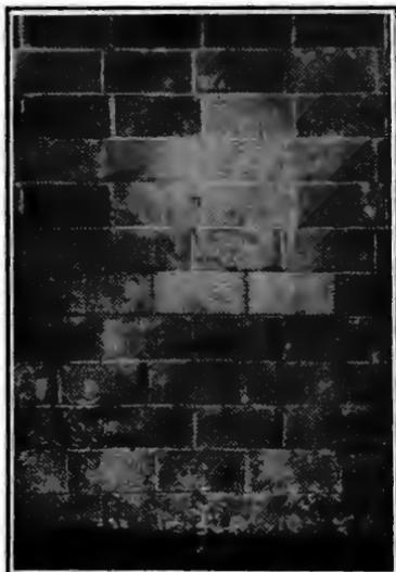
Fig. 13. The lower courses are double wall construction and the upper single wall construction.
