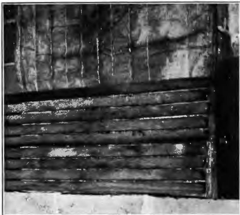
Fig. 25. A method of applying insulating quilt and lath.
