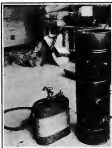
Fig. 9. Oil tank and spray pump for oiling forms.
