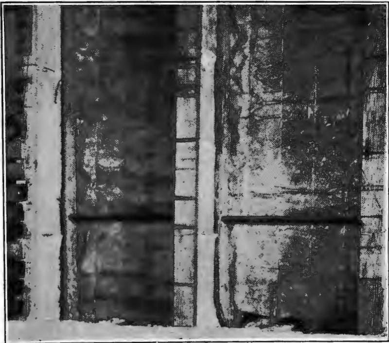
Fig. 24. One method of applying insulating quilt between studs.
