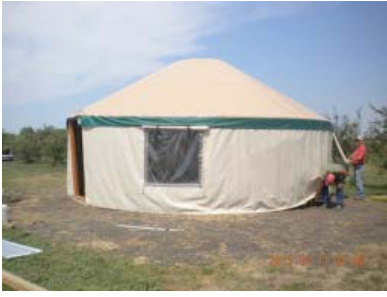
The yurt kit that was used included three windows in the side walls.
