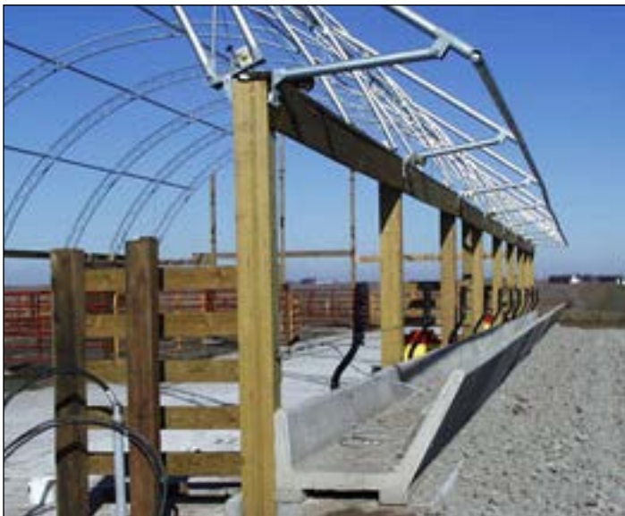
A feed bunk is placed outside of the wall to eliminate the expense of an interior drive alley. An overhang is added to reduce the rainwater entering the bunk. It is calculated for one foot of feed bunk per head.
