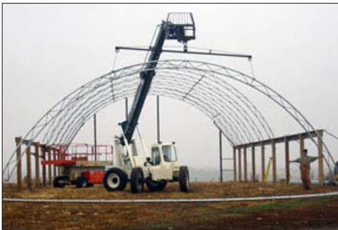
Hoop barns are constructed using steel arches mounted on wood or concrete sidewalls.
