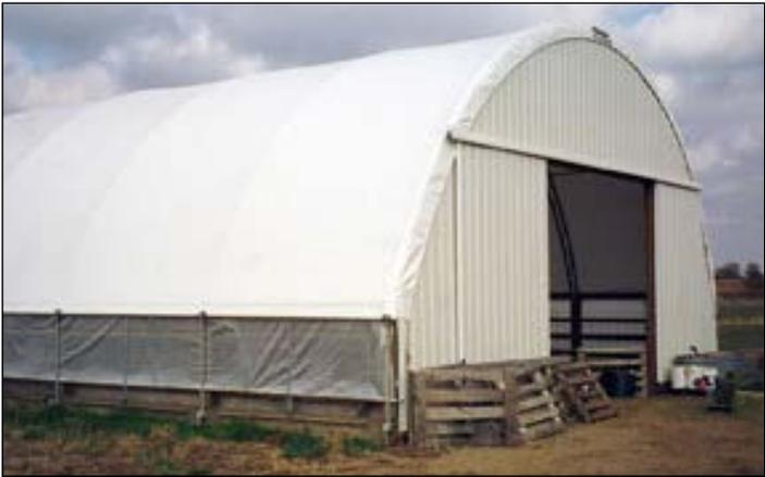
Sheep tend to thrive in cool but dry environments which hoop barns can provide when they are well-ventilated. Sidewall curtains and end wall openings help to promote good ventilation, thereby keeping the humidity and ammonia to minimum levels, which is important for animal comfort and health.
