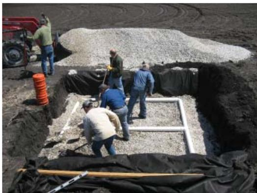
*Members of the SFWA assisting in the installation of a blind inlet. In this image the drain pipe has been installed and connected to the riser and is being covered with gravel.*
